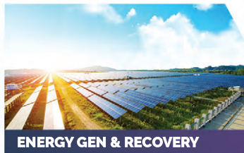
ENERGY GEN & RECOVERY
